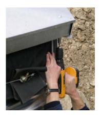
9. The structure is completed by the addition of the disc apex cover to the top hub plate, securing it into position with the bolt provided.
