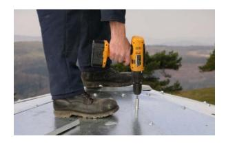
Speed bit complete with <u>13mm</u> socket
