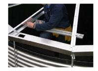
8. Remove the access hatches from their associated sheets and place one over the segment designated for water inlet. You will notice that the segment sheets are folded along the left hand edge and that the holes on that side are slotted. Position the sheet and place two M8 bolts in the right hand holes to keep it in position.
