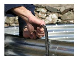
2. Roll out the liner over the 50mm sand base, laying it out so that the base to wall circumference seam is touching the steelwork all around. The vertical side will then be laying flat on the base. BEFORE working with the liner check the sand for stones or sharp objects. Also check your SHOES.
