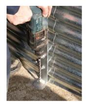
'PODGER' or strong screwdriver to align and hold the steel panels
