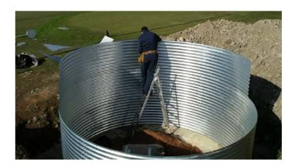
It is essential that each alternate ring is staggered i.e. the end of each panel should rest towards the middle of the panels below, similar to a brickwork effect.
